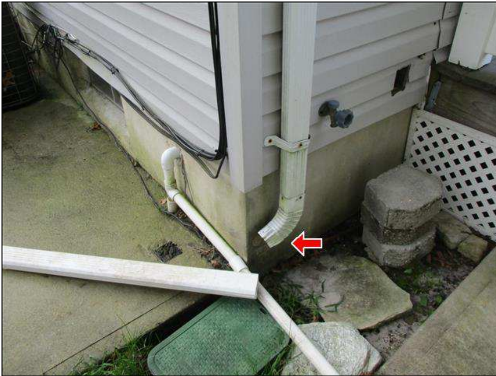
1.3 Item 1(Picture) Gutter downspout termination
