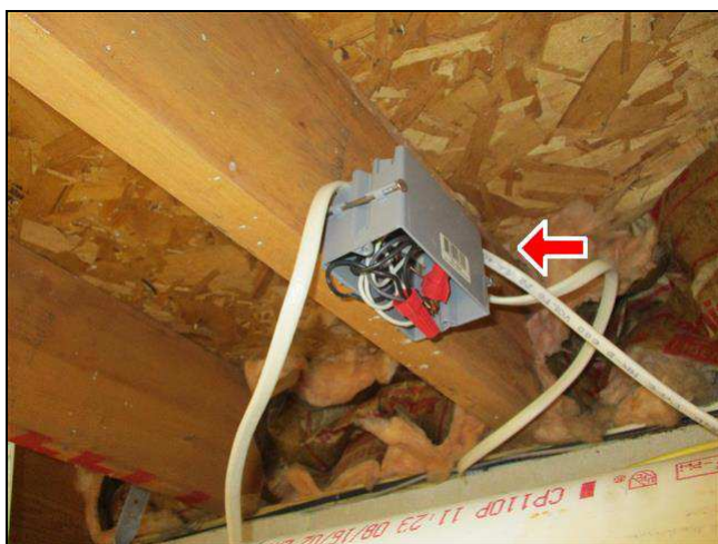
6.3 Item 2(Picture) Basement junction box
