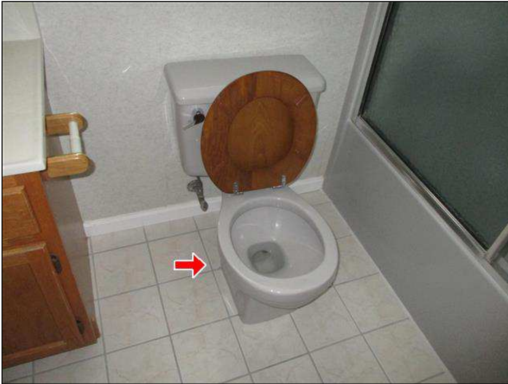
5.0 Item 1(Picture) Loose toilet
