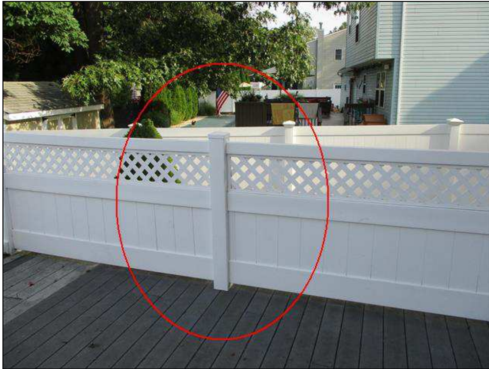
2.3 Item 3(Picture) Loose handrail
