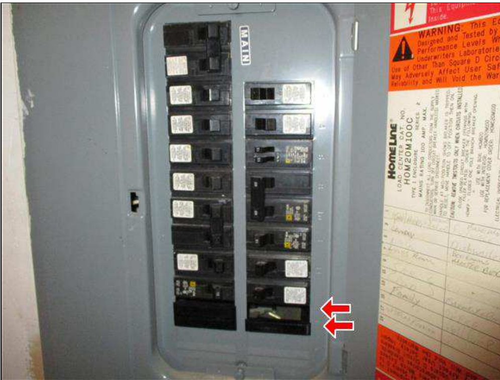
6.1 Item 2(Picture) Missing knockout covers
