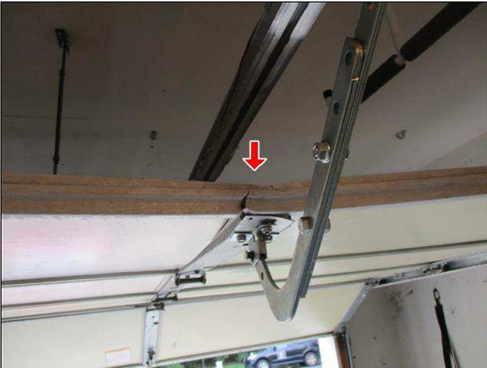
9.3 Item 1(Picture) Garage door
