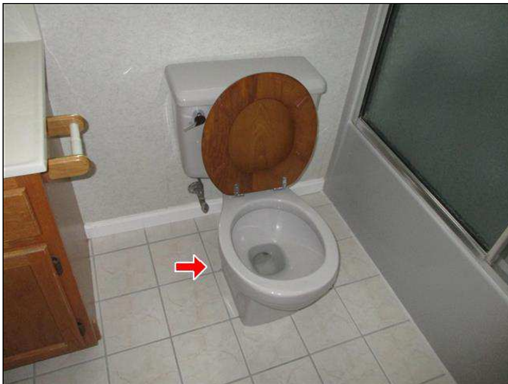
5.0 Item 1(Picture) Loose toilet
