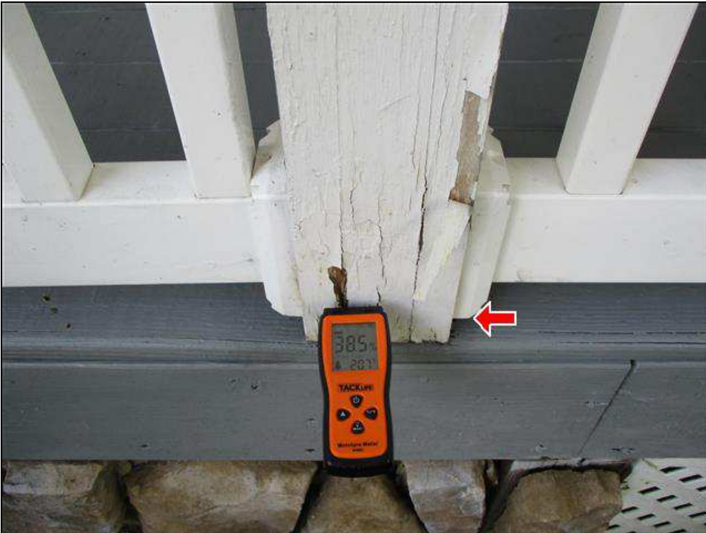
2.3 Item 4(Picture) Deck railing post
