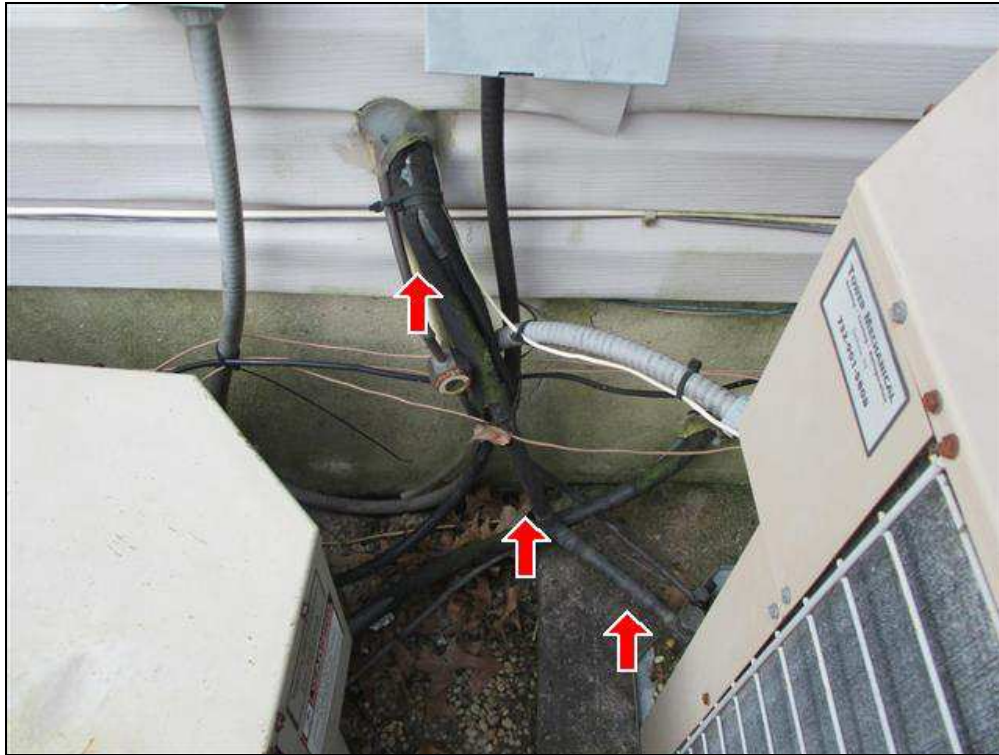
4.8 Item 1(Picture) Missing insulation
