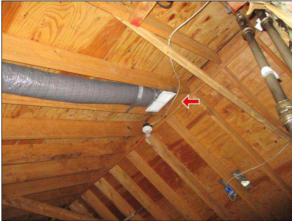
4.3 Item 1(Picture) Supply duct in attic
