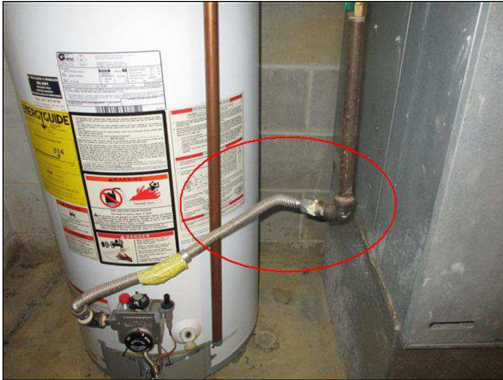
5.2 Item 2(Picture) No drip leg
