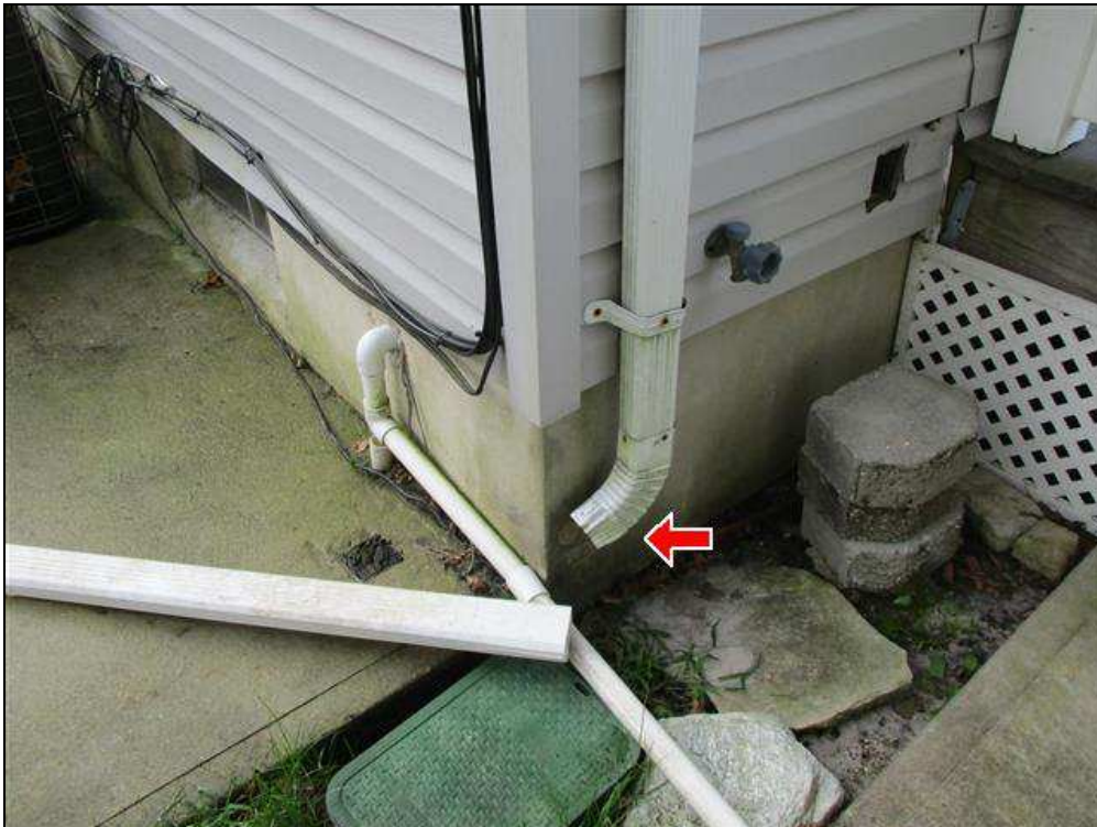
1.3 Item 1(Picture) Gutter downspout termination
