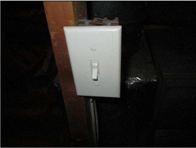
4.2 Item 1(Picture) Emergency shut off switch (attic furnace)
