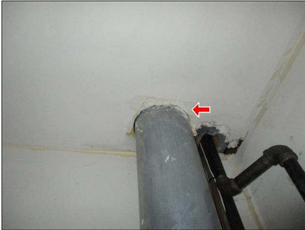
4.5 Item 1(Picture) Water heater and furnace chimney
