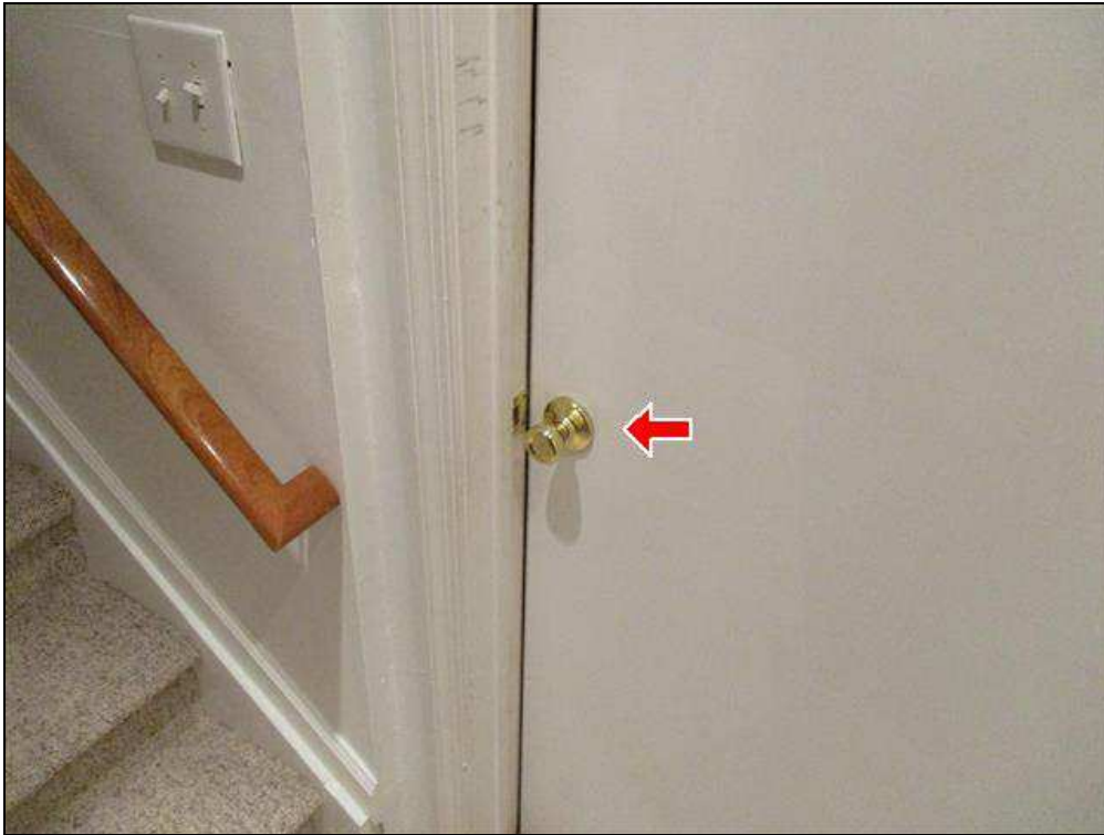
8.5 Item 1(Picture) Basement office
