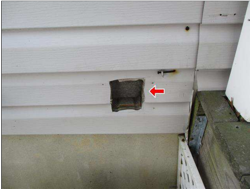
2.0 Item 1(Picture) Hole in siding
