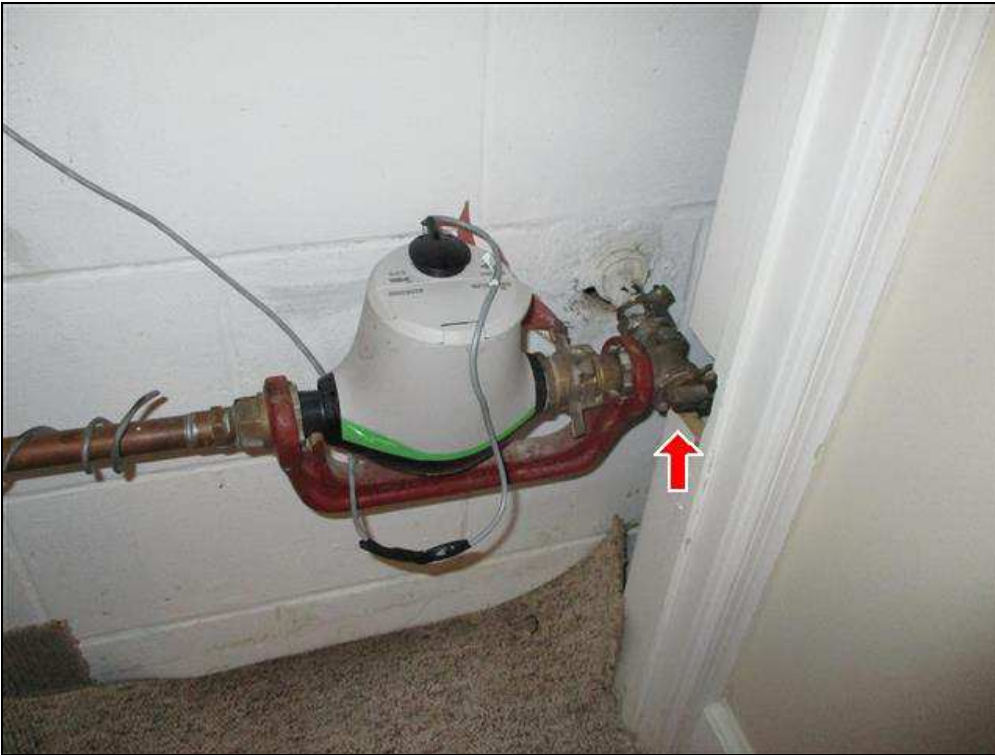
5.3 Item 1(Picture) Main water shut off
