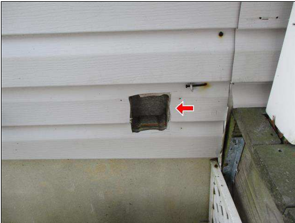
2.0 Item 1(Picture) Hole in siding
