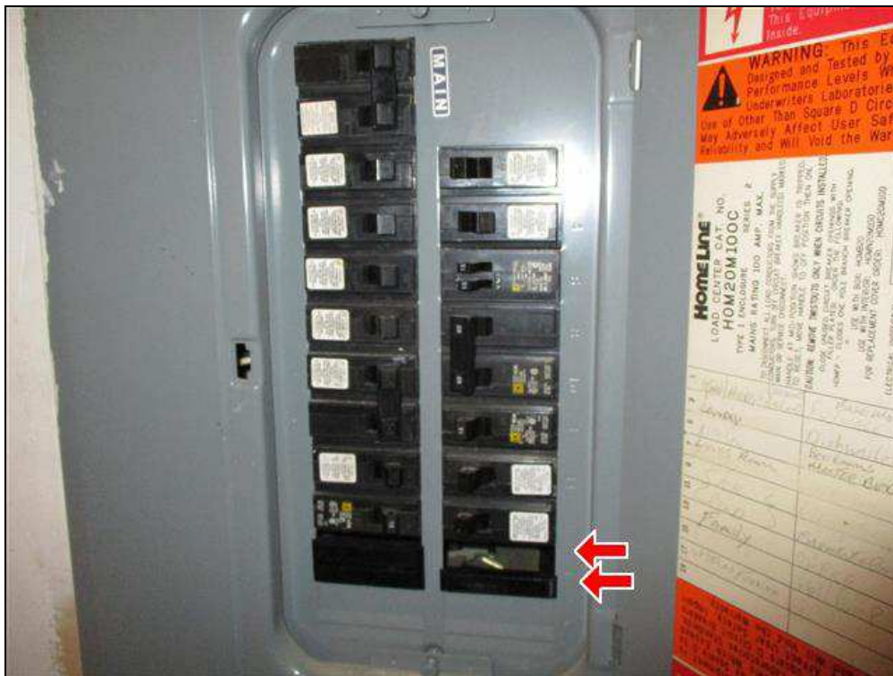
6.1 Item 2(Picture) Missing knockout covers
