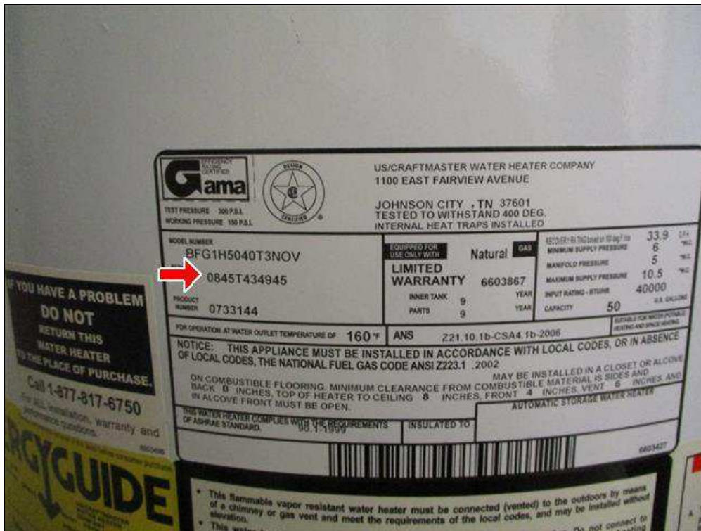
5.2 Item 1(Picture) Water heater data plate
