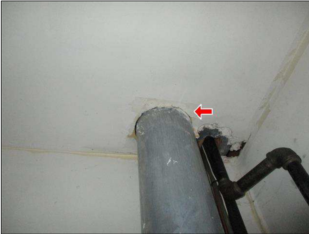
4.5 Item 1(Picture) Water heater and furnace chimney
