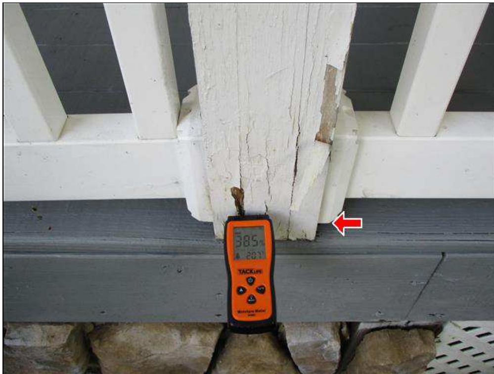
2.3 Item 4(Picture) Deck railing post
