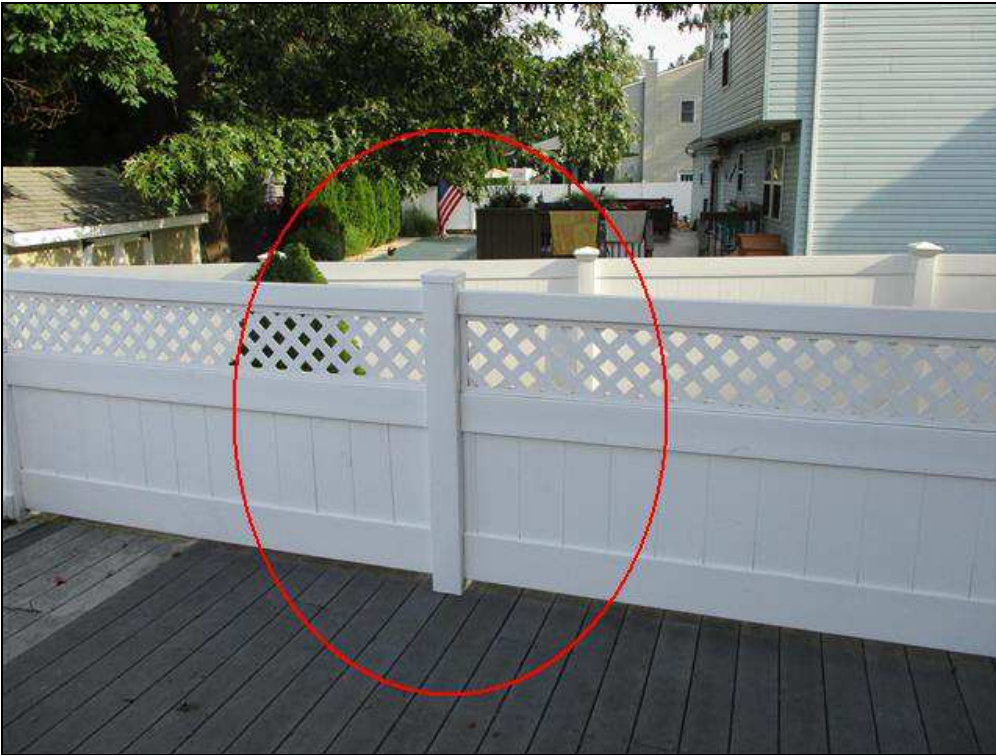
2.3 Item 3(Picture) Loose handrail
