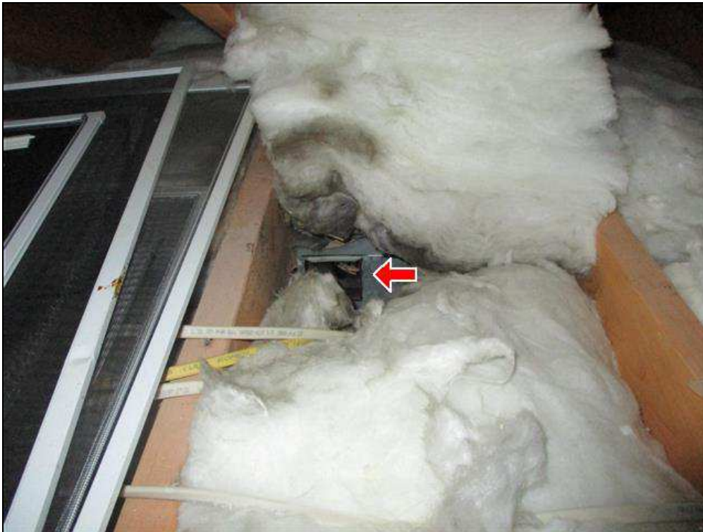
7.4 Item 1(Picture) Master bathroom exhaust fan
