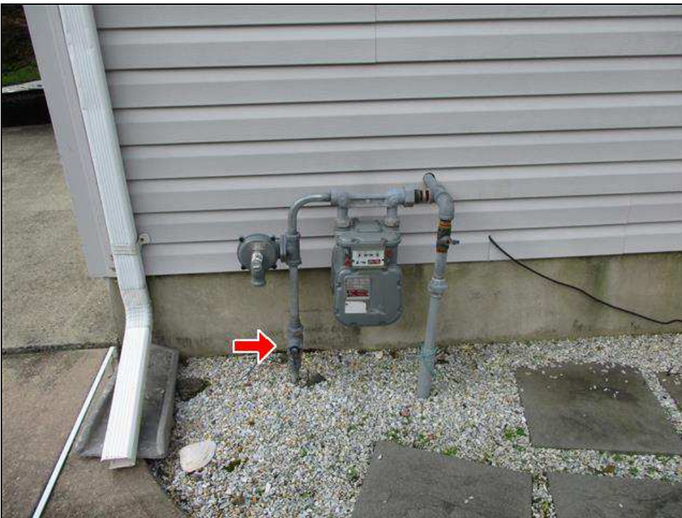
5.5 Item 1(Picture) Main gas shut off
