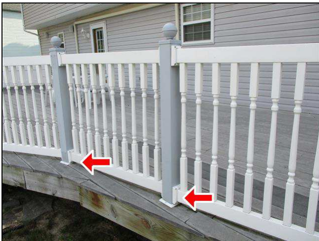
2.3 Item 2(Picture) Loose handrail
