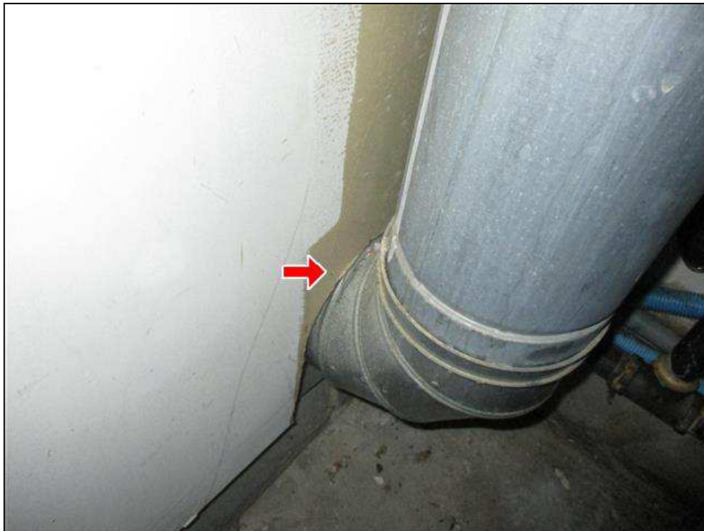
4.5 Item 2(Picture) Water heater and furnace chimney
