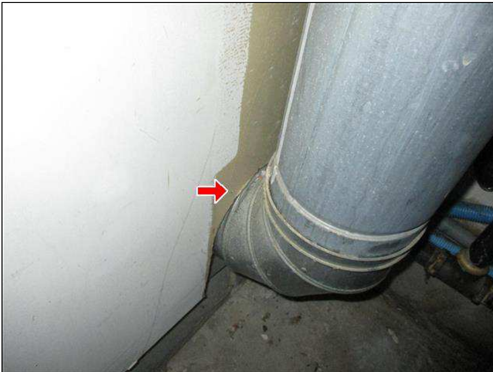
4.5 Item 2(Picture) Water heater and furnace chimney
