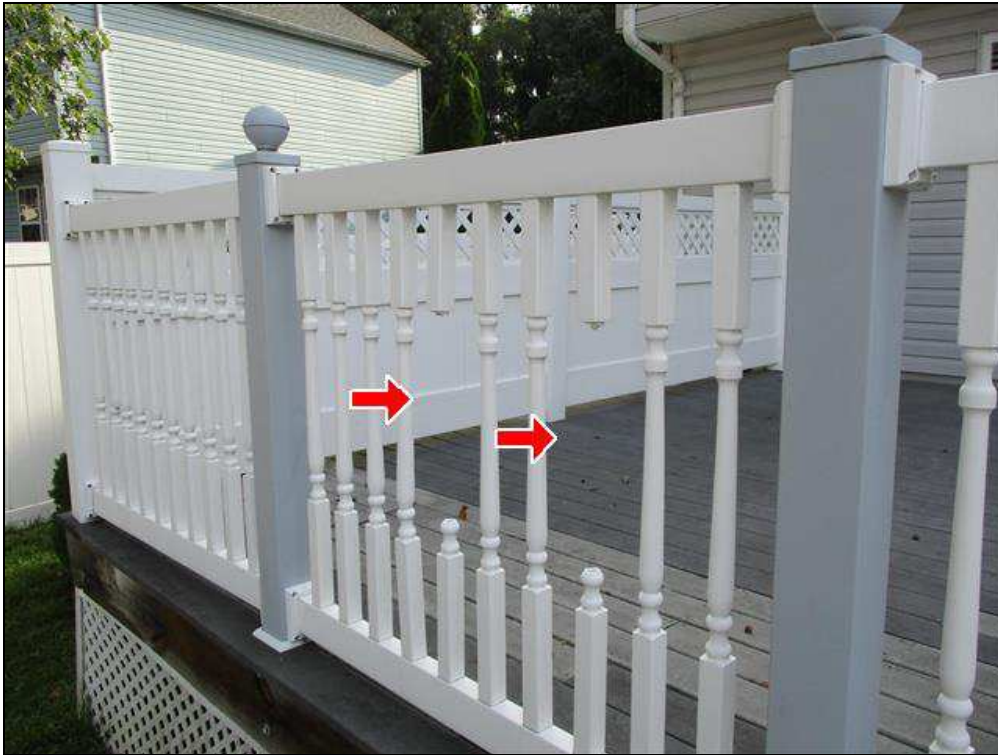
2.3 Item 1(Picture) Missing spindles
