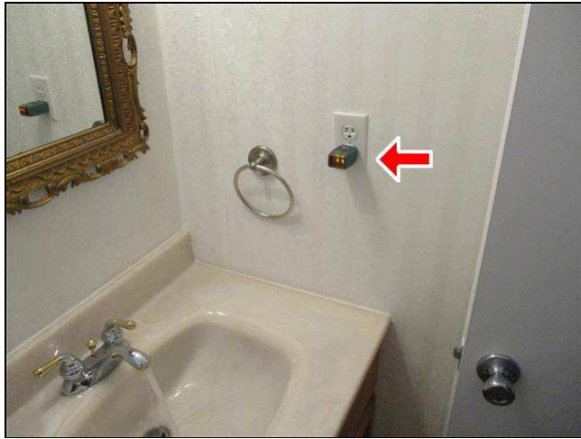
6.4 Item 1(Picture) First floor bathroom
