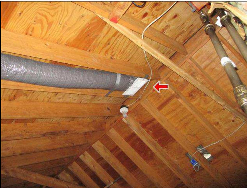
4.3 Item 1(Picture) Supply duct in attic
