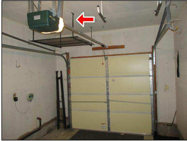
9.5 Item 1(Picture) Garage door operator
