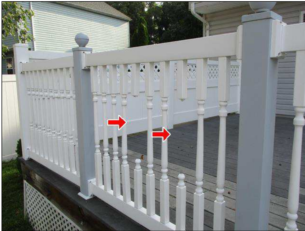
2.3 Item 1(Picture) Missing spindles
