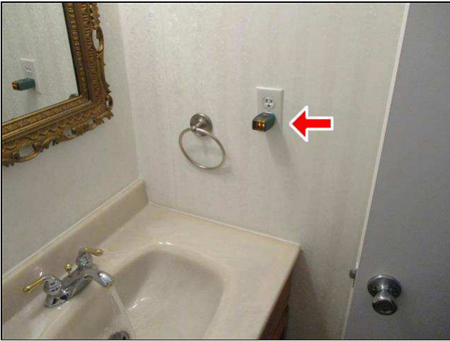
6.4 Item 1(Picture) First floor bathroom
