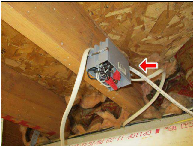
6.3 Item 2(Picture) Basement junction box
