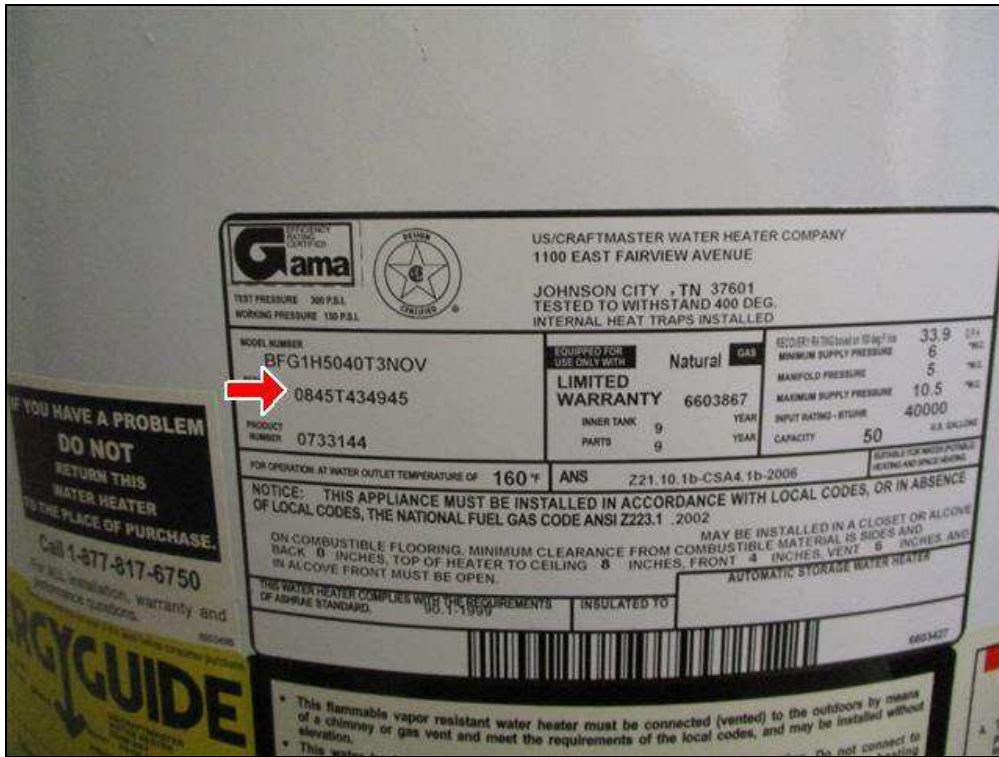
5.2 Item 1(Picture) Water heater data plate
