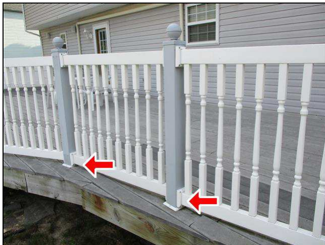
2.3 Item 2(Picture) Loose handrail
