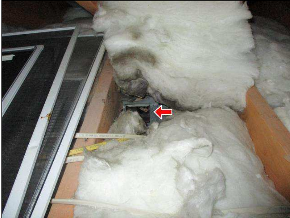
7.4 Item 1(Picture) Master bathroom exhaust fan
