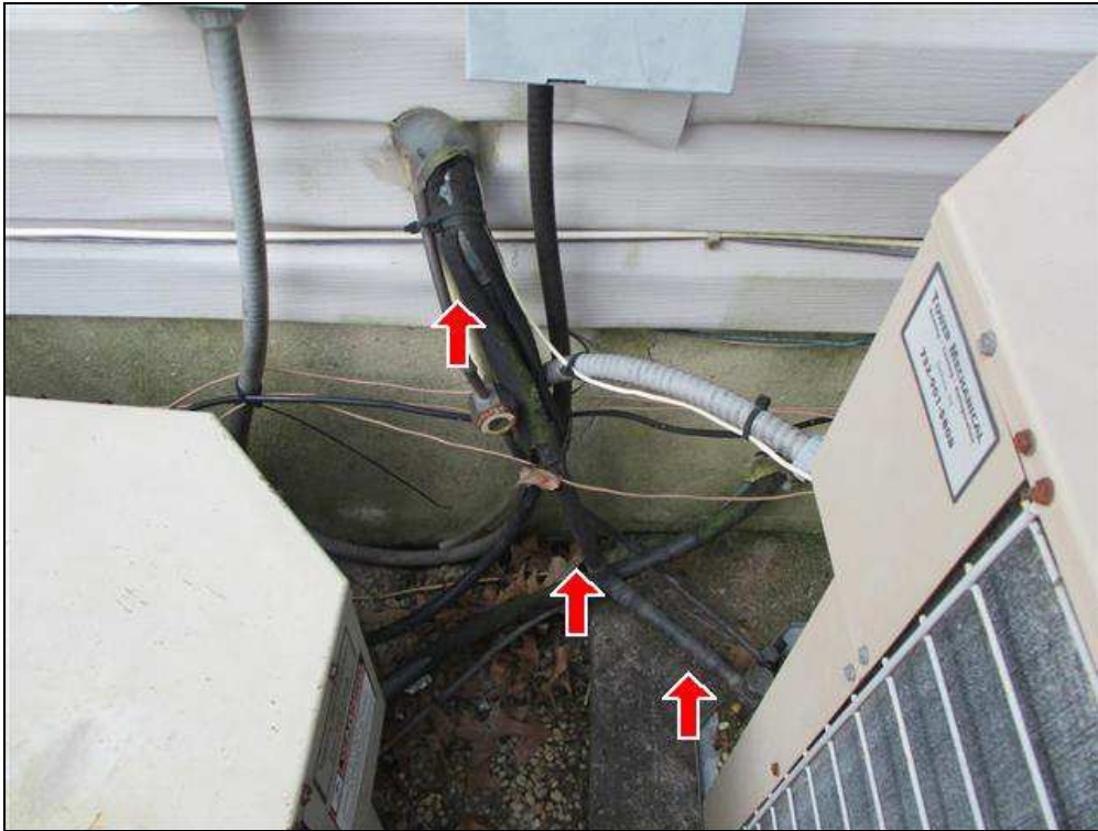
4.8 Item 1(Picture) Missing insulation
