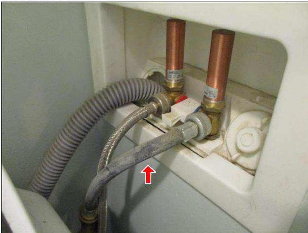
5.1 Item 2(Picture) Clothes washer supply hoses
