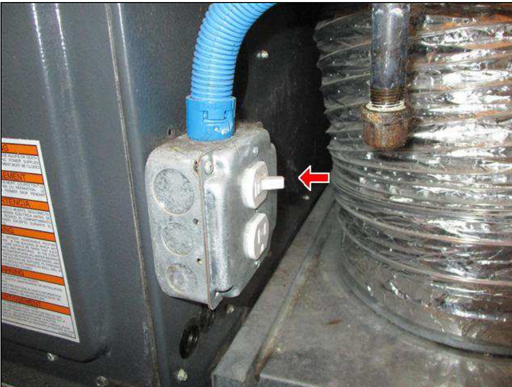
4.2 Item 2(Picture) Emergency shut off at lower level furnace
