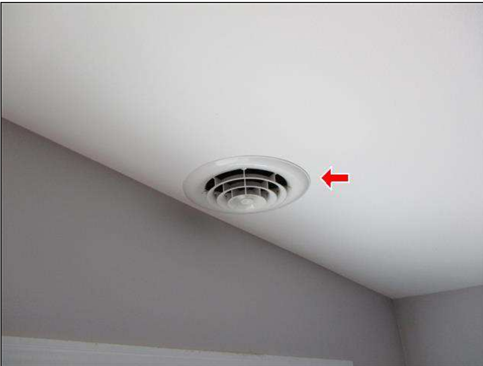
4.3 Item 2(Picture) Master bedroom supply duct
