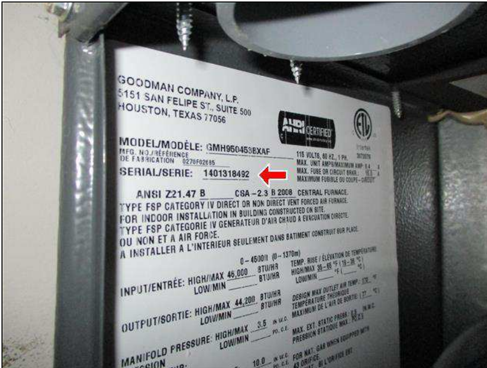
4.0 Item 2(Picture) Furnace data plate (lower level)
