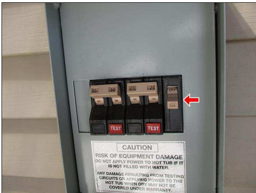
6.7 Item 2(Picture) Sub panel
