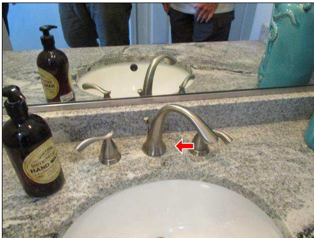
5.1 Item 1(Picture) Hallway bathroom sink
