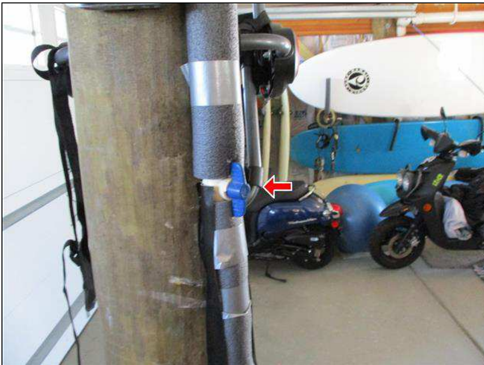
5.3 Item 1(Picture) Main water shut off
