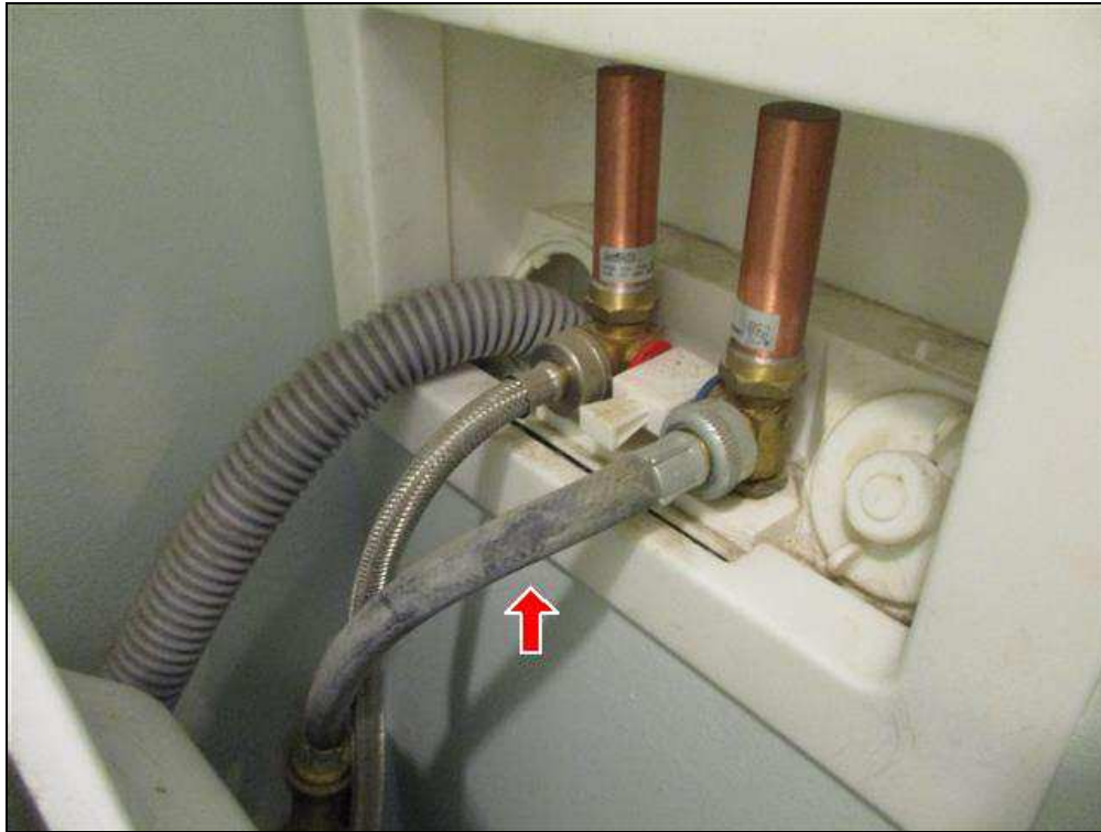
5.1 Item 2(Picture) Clothes washer supply hoses
