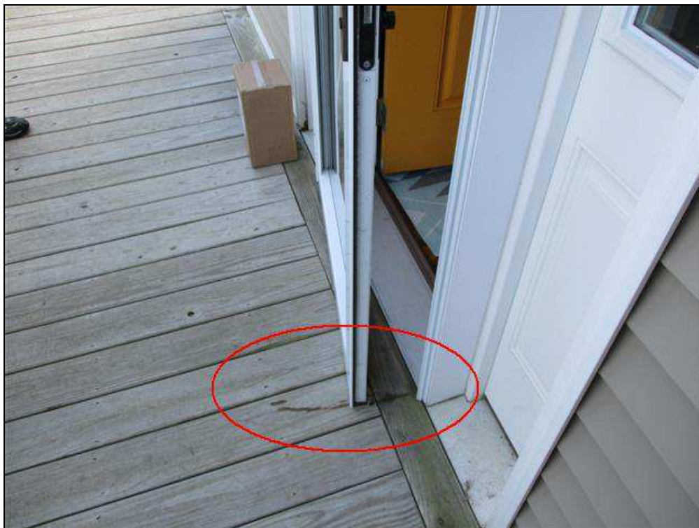
2.1 Item 1(Picture) Storm door
