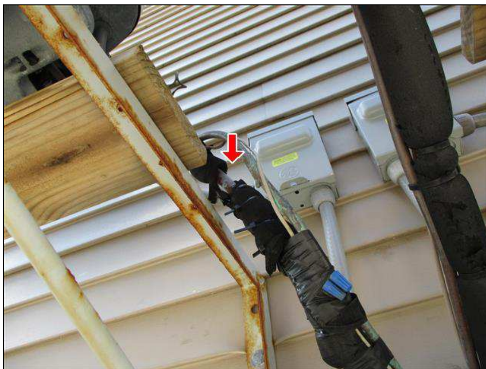
4.8 Item 2(Picture) Missing insulation
