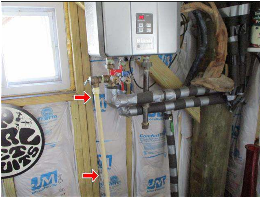
5.2 Item 1(Picture) TPRV valve
