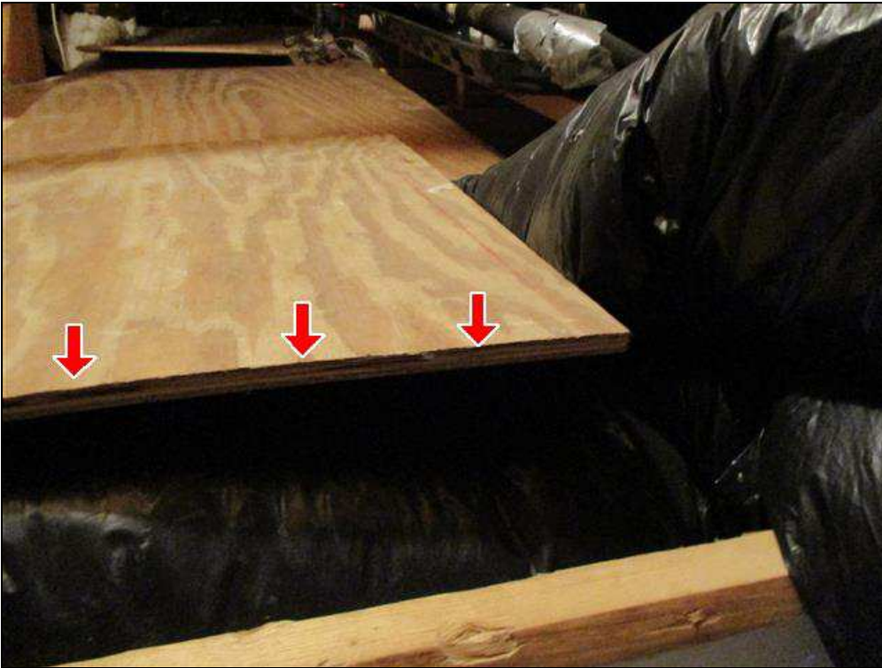
4.3 Item 1(Picture) Supply duct leading to master bedroom
