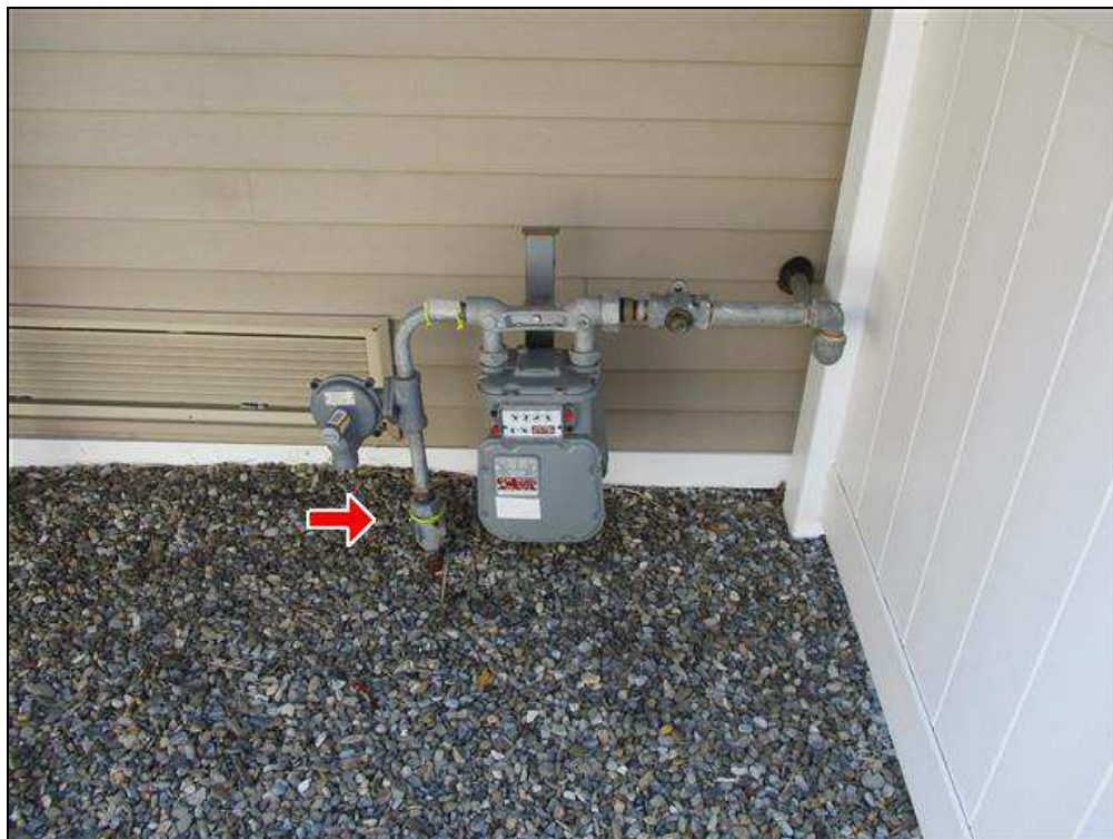
5.5 Item 1(Picture) Main gas shut off
