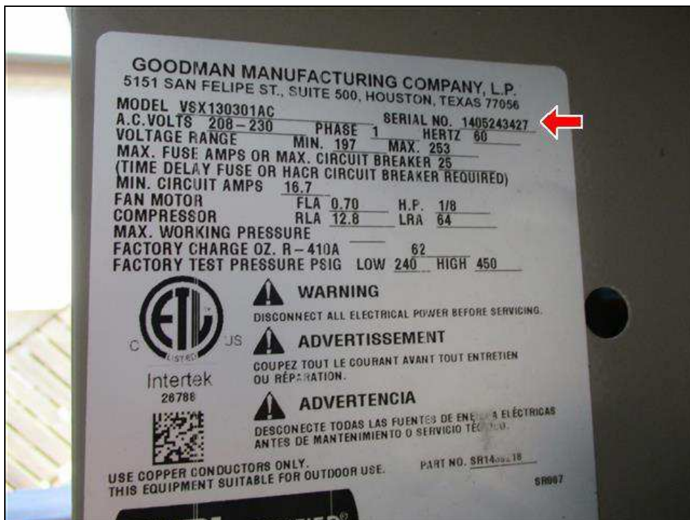
4.8 Item 1(Picture) A/C condensing unit data plate
