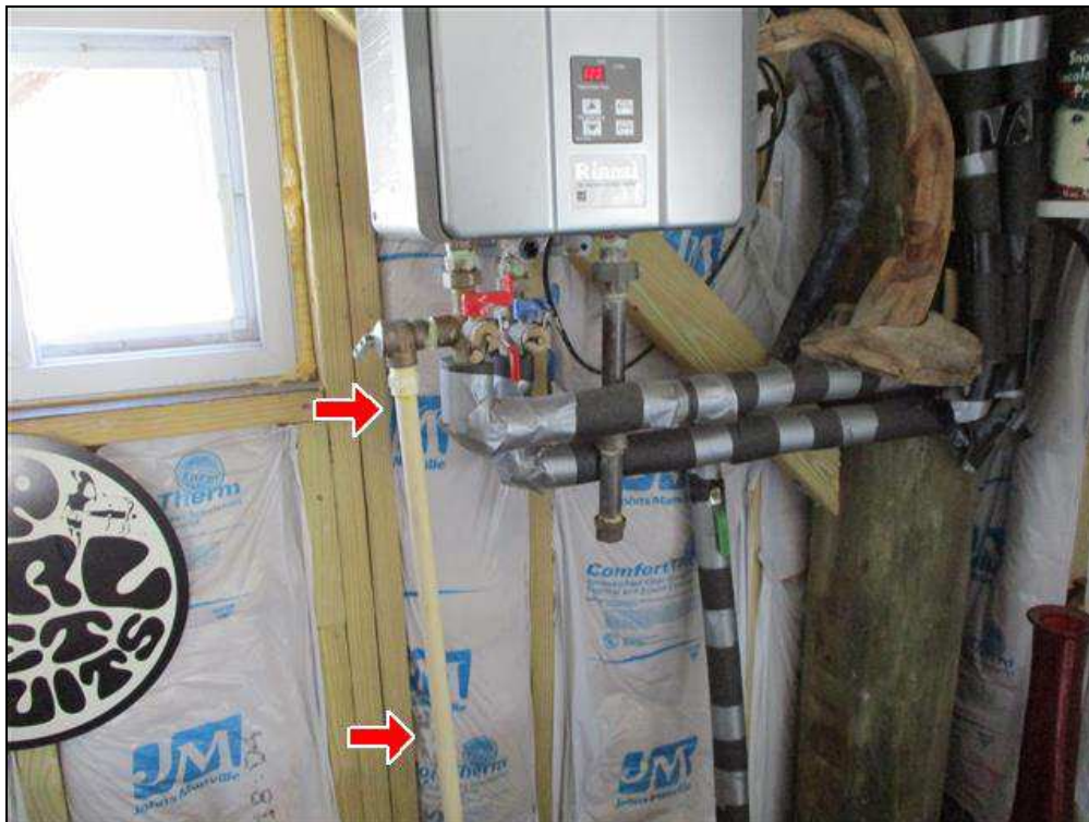
5.2 Item 1(Picture) TPRV valve
