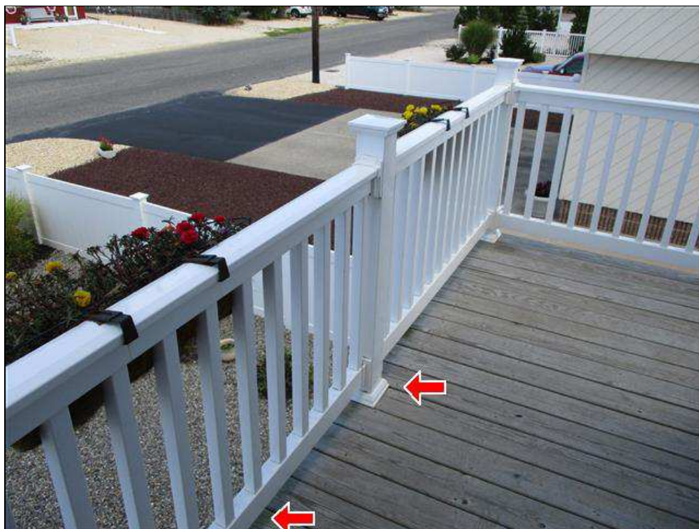
2.3 Item 2(Picture) Front handrail
