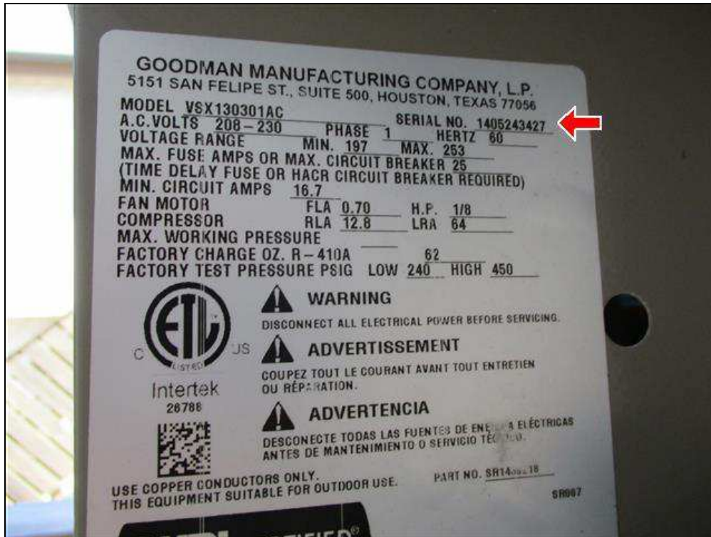
4.8 Item 1(Picture) A/C condensing unit data plate
