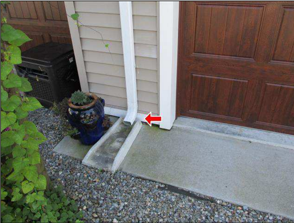
1.3 Item 2(Picture) Gutter downspout termination
