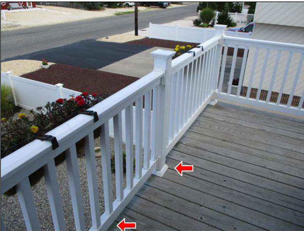
2.3 Item 2(Picture) Front handrail
