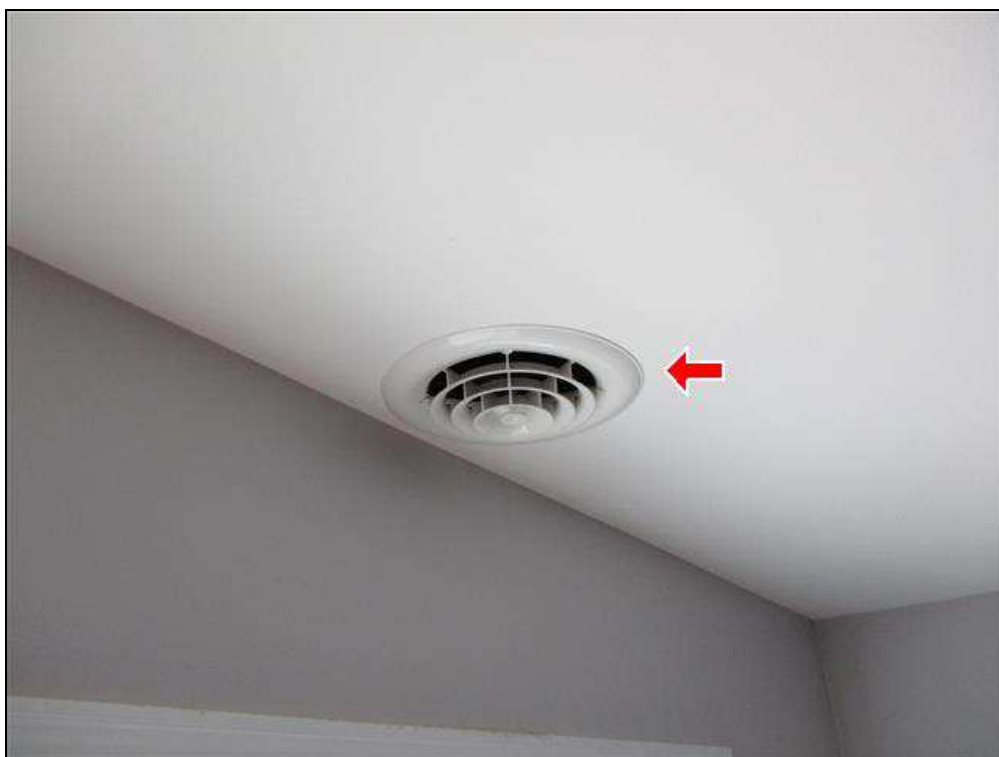
4.3 Item 2(Picture) Master bedroom supply duct
