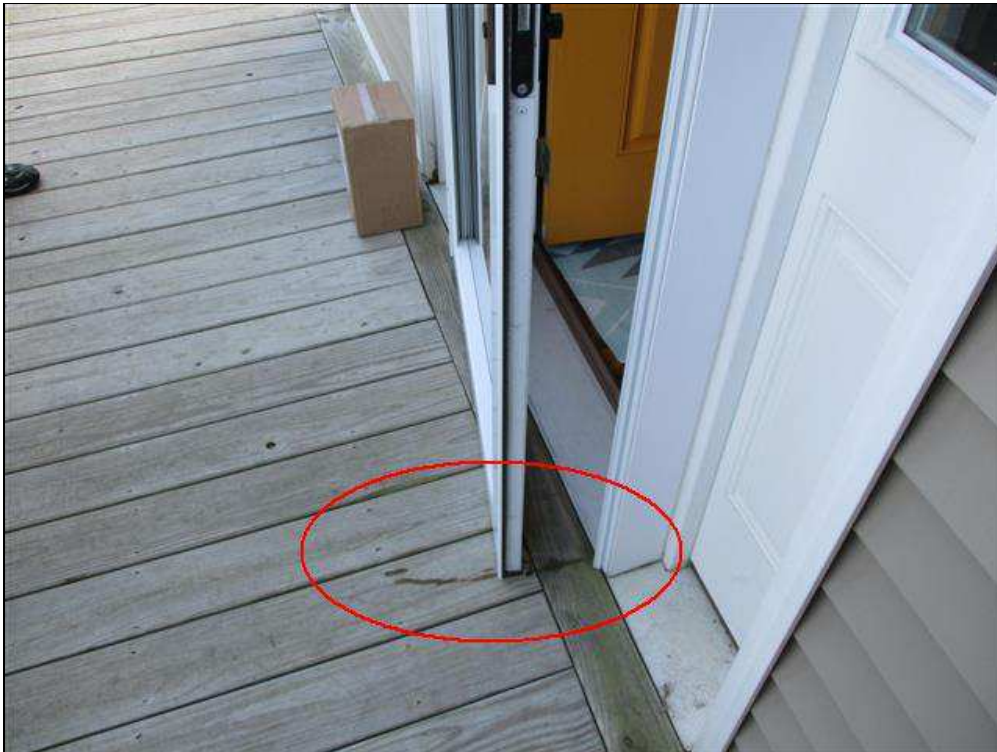
2.1 Item 1(Picture) Storm door
