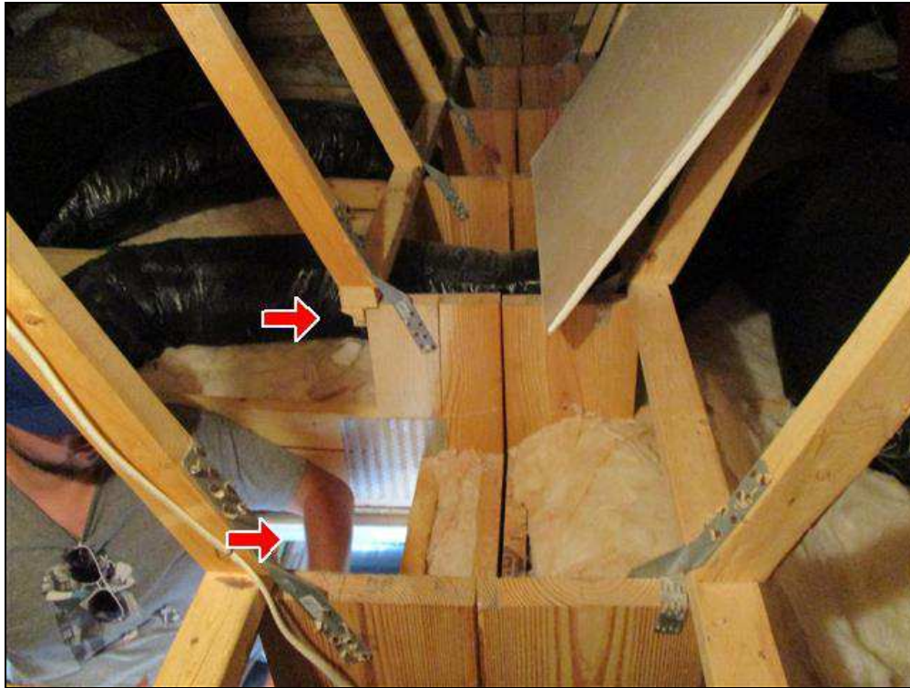
3.5 Item 1(Picture) Cut roof truss
