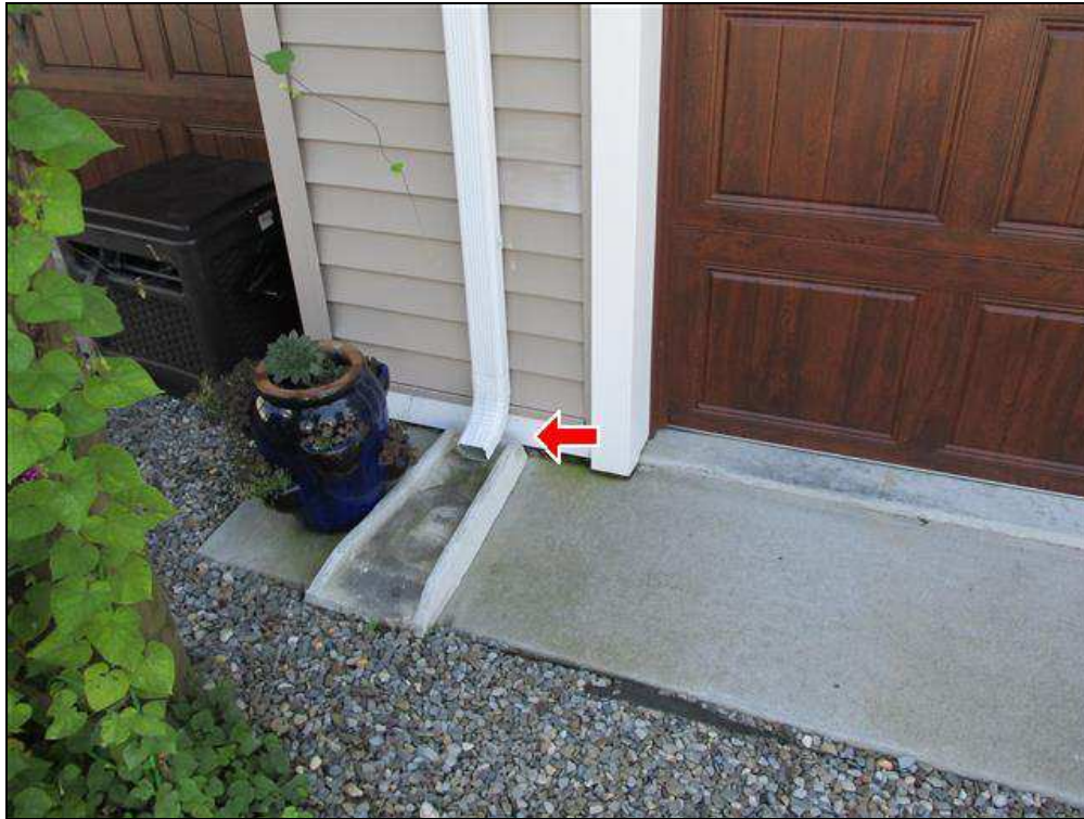
1.3 Item 2(Picture) Gutter downspout termination
