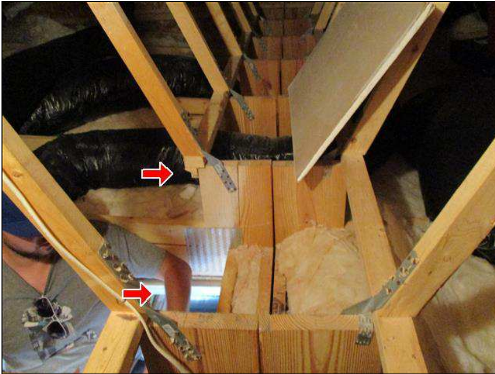
3.5 Item 1(Picture) Cut roof truss
