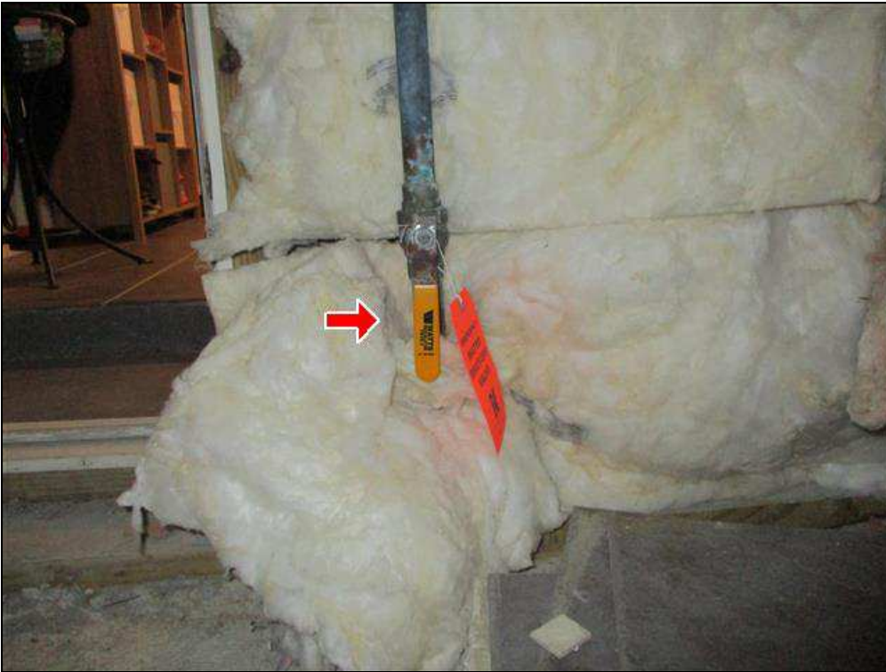
5.3 Item 1(Picture) Main water shut off
