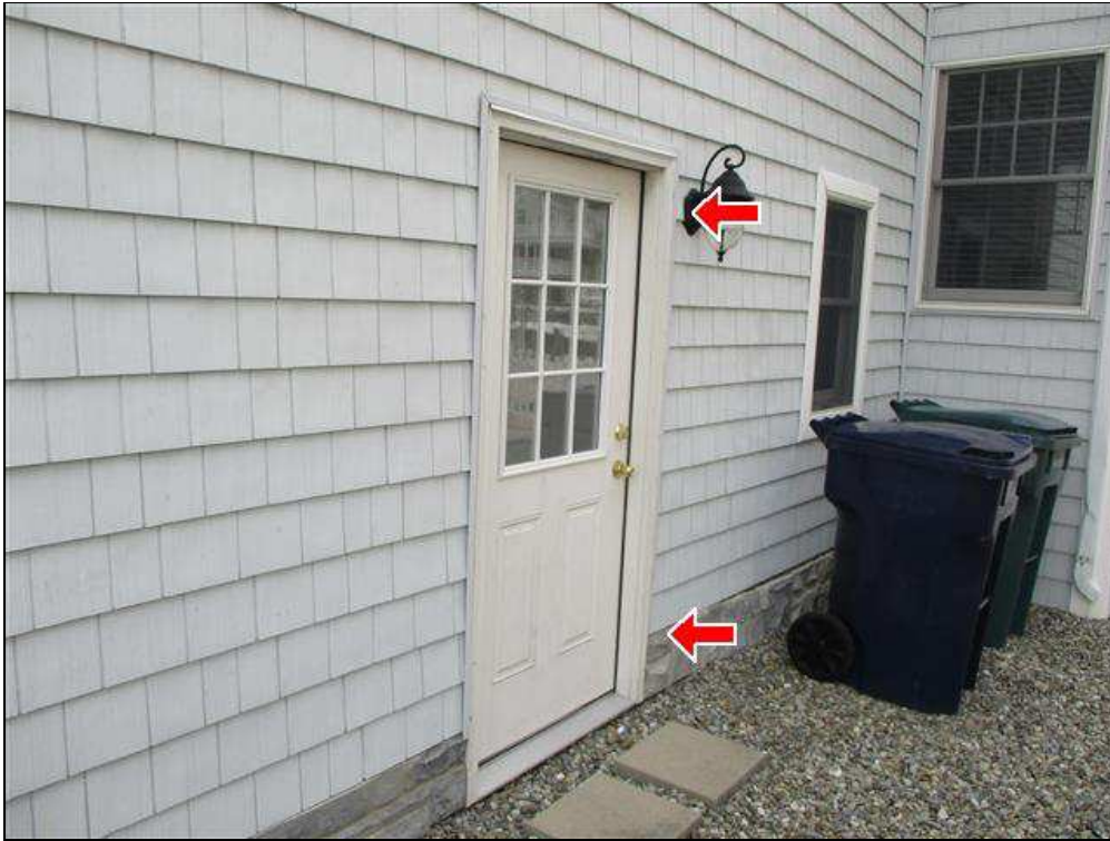
2.1 Item 1(Picture) Garage entry door
