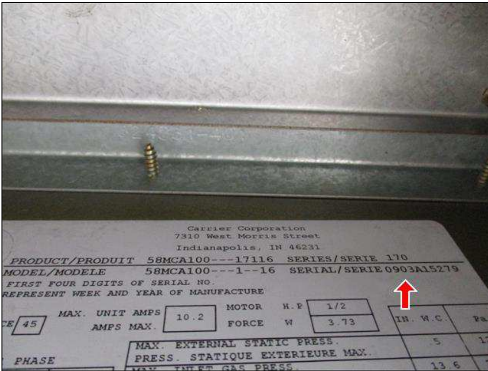
4.0 Item 1(Picture) Furnace data plate (garage unit)
