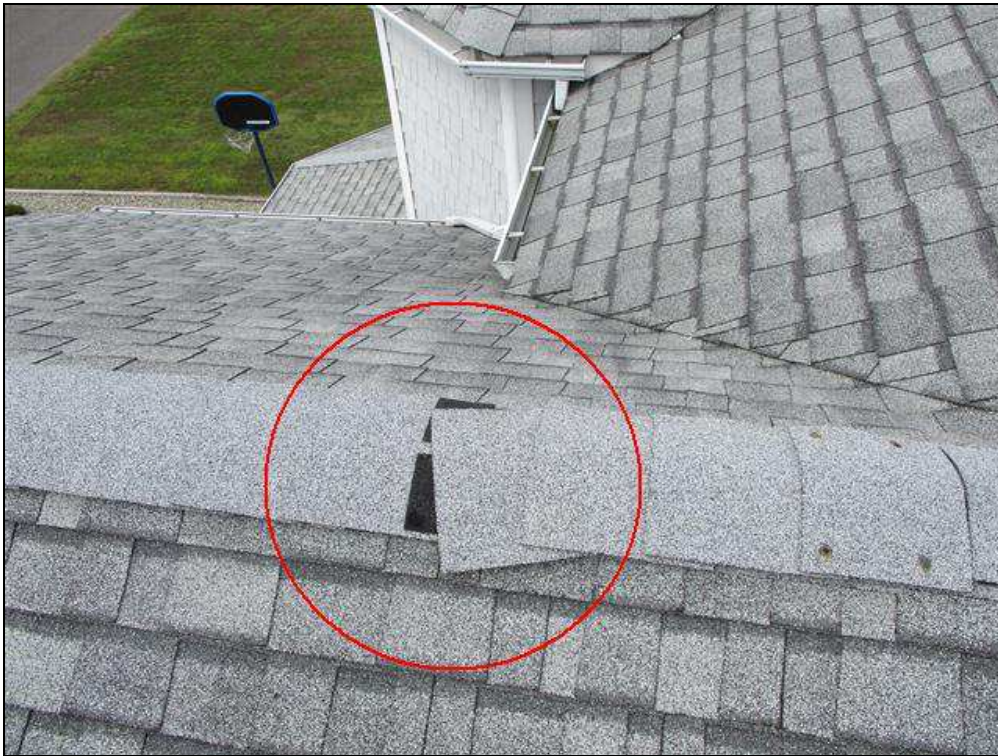
1.0 Item 1(Picture) Loose roof shingle
