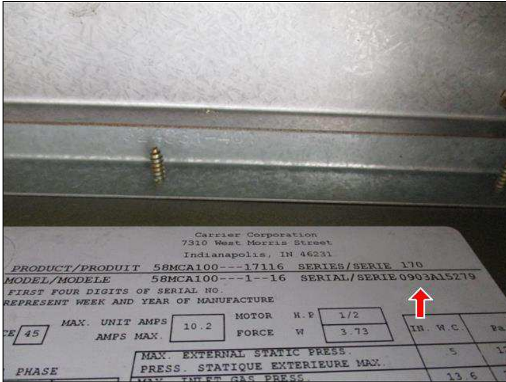
4.0 Item 1(Picture) Furnace data plate (garage unit)
