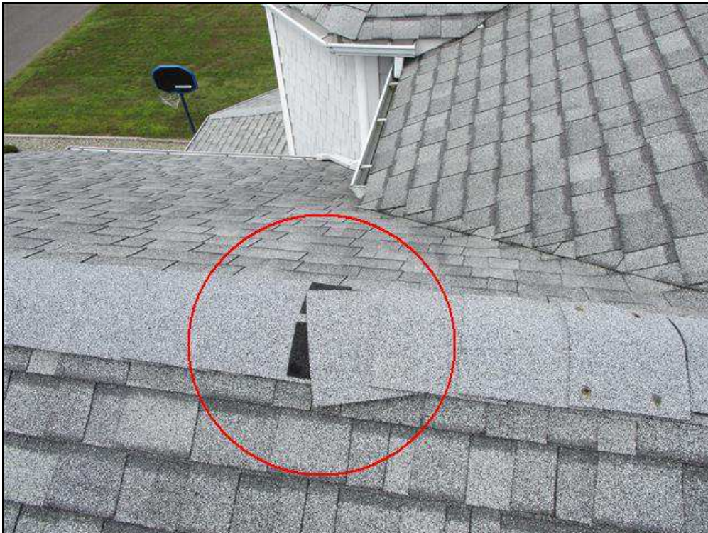
1.0 Item 1(Picture) Loose roof shingle
