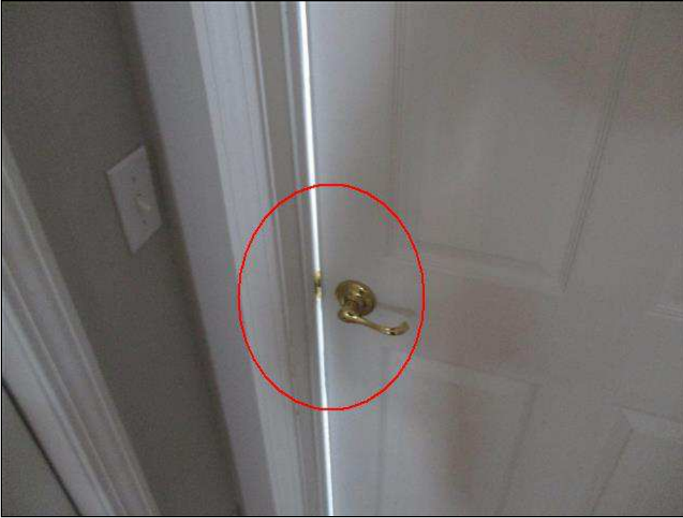
8.5 Item 1(Picture) Master bedroom door
