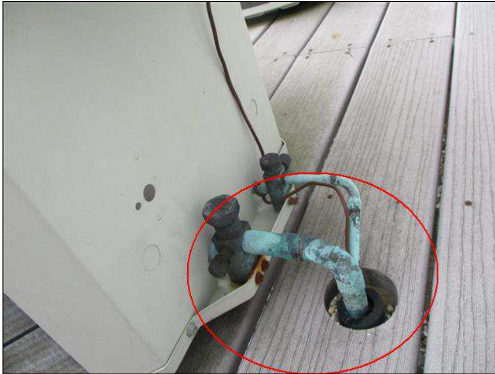
4.8 Item 2(Picture) Missing insulation
