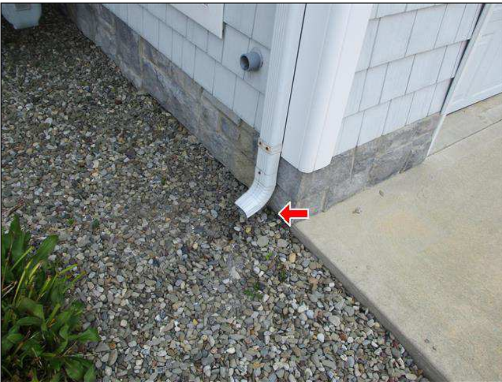
1.3 Item 1(Picture) Gutter downspout termination
