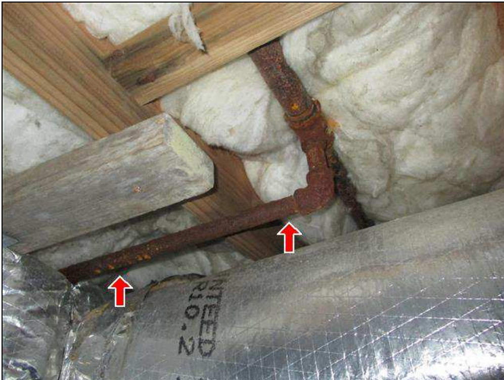
5.4 Item 1(Picture) Gas lines
