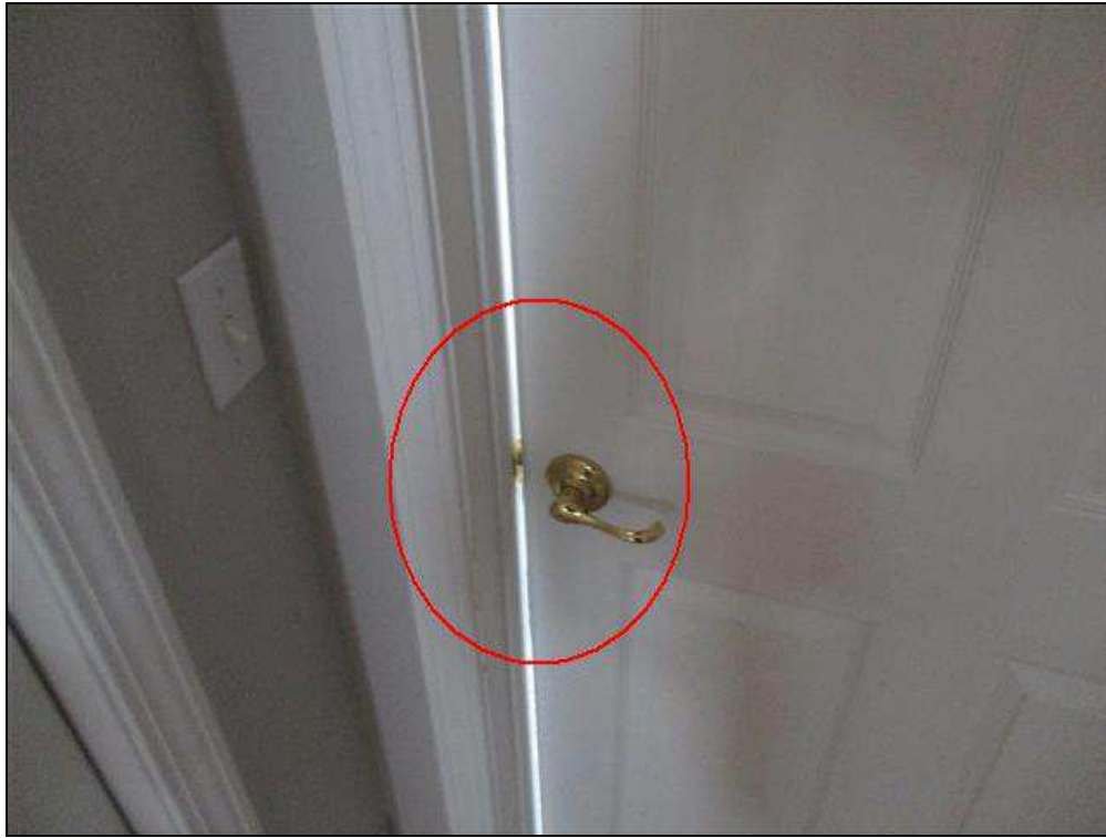
8.5 Item 1(Picture) Master bedroom door
