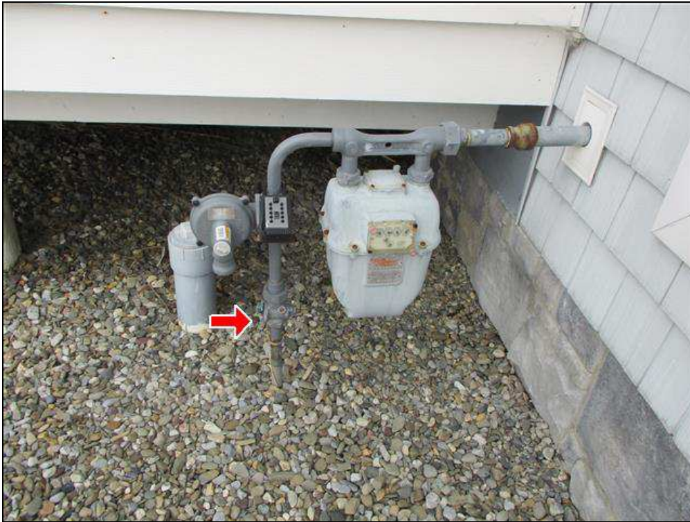
5.5 Item 1(Picture) Main fuel shut off
