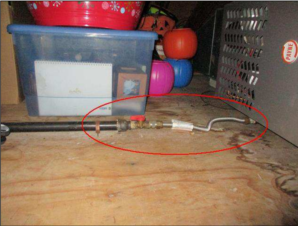
4.0 Item 6(Picture) No drip leg
