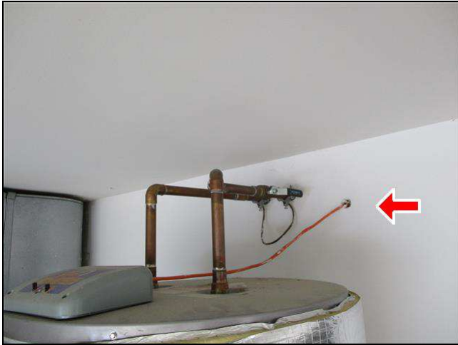
5.2 Item 1(Picture) Water heater
