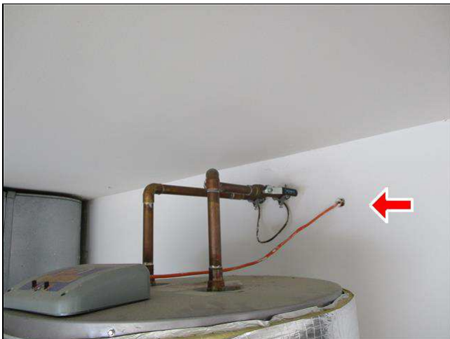
5.2 Item 1(Picture) Water heater
