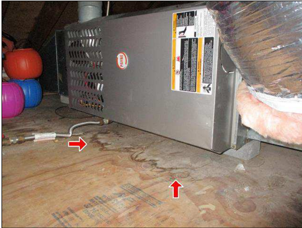
4.0 Item 3(Picture) No secondary condensate drain pan (attic unit)
