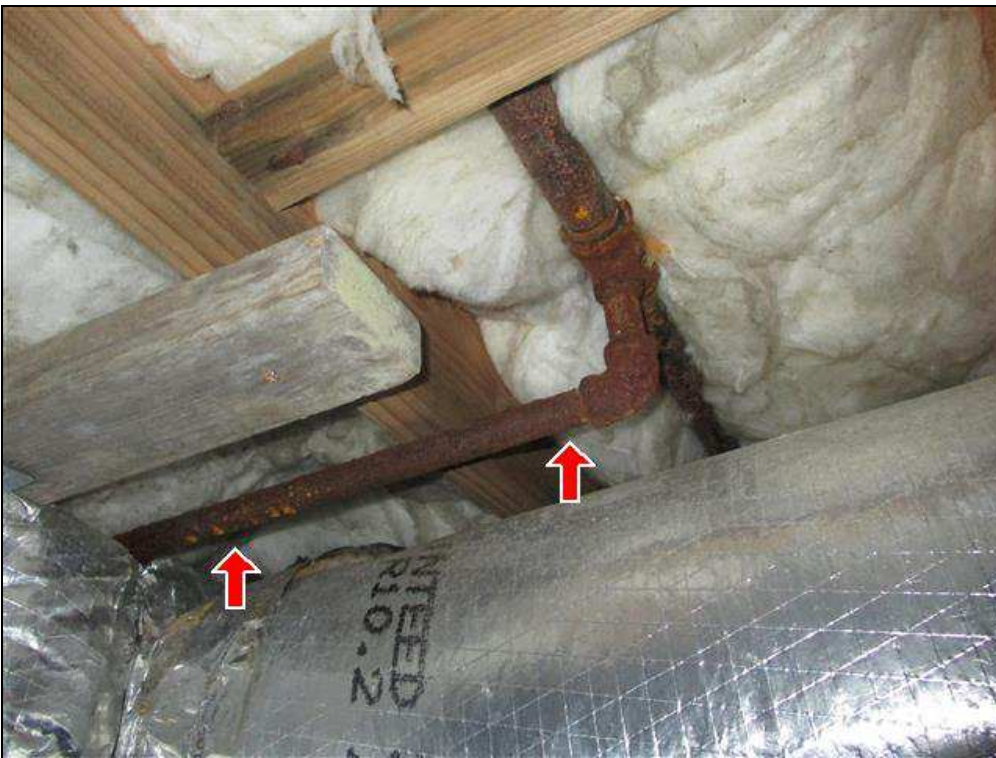
5.4 Item 1(Picture) Gas lines
