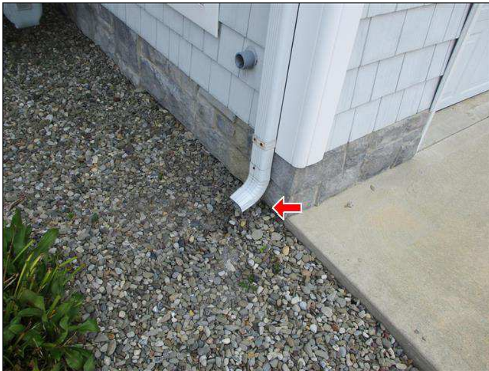
1.3 Item 1(Picture) Gutter downspout termination
