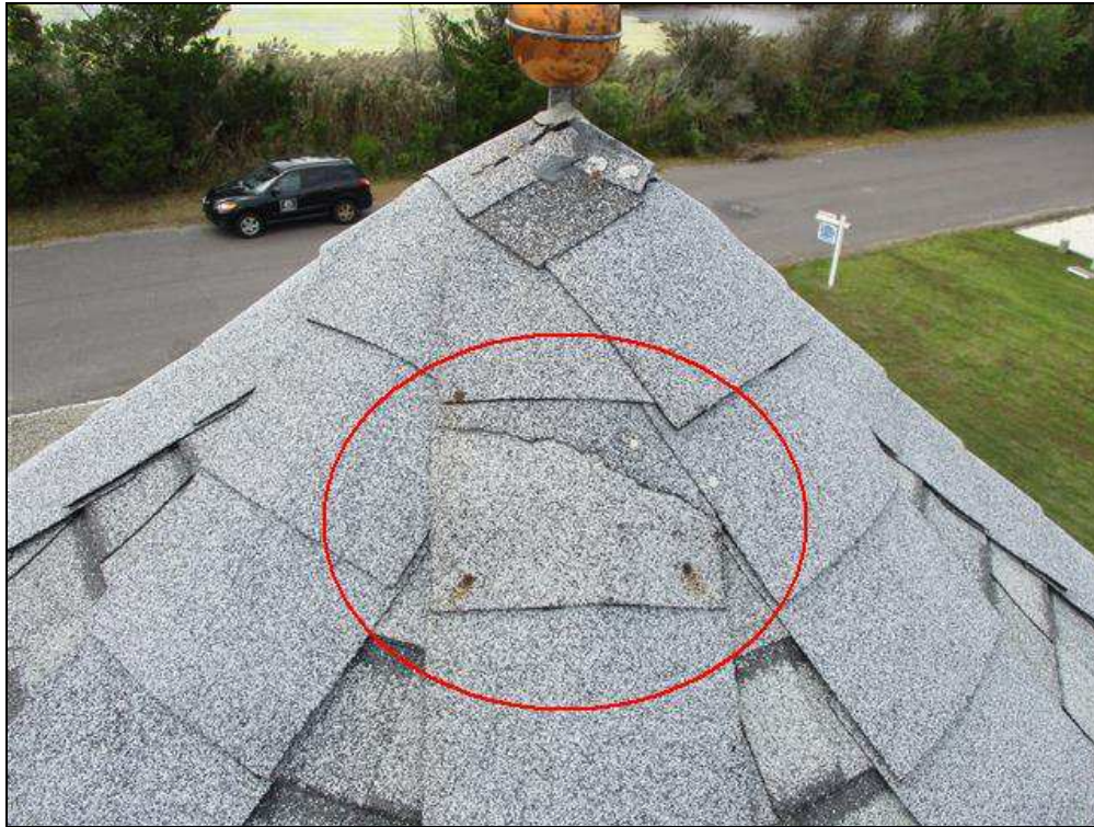
1.0 Item 2(Picture) Damaged roof shingle
