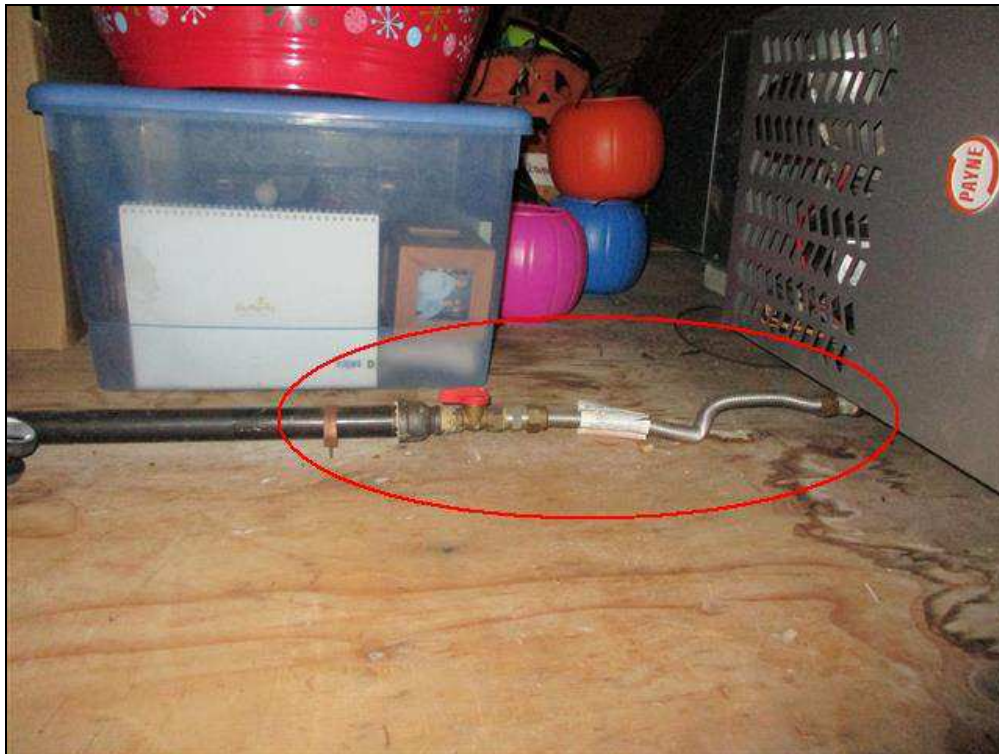
4.0 Item 6(Picture) No drip leg
