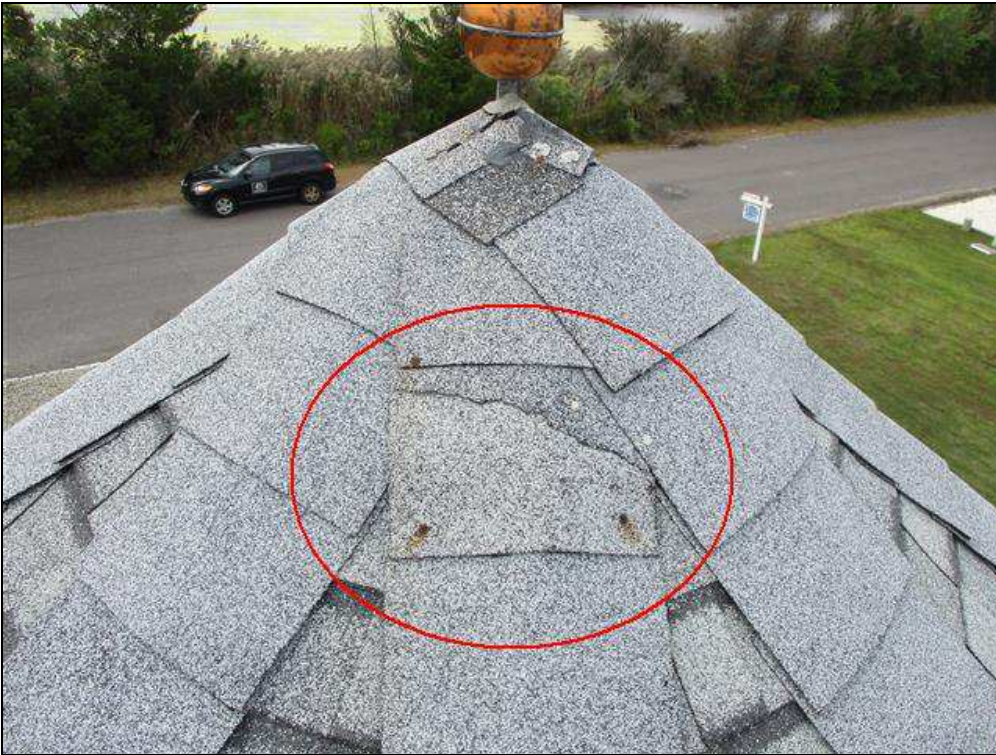
1.0 Item 2(Picture) Damaged roof shingle
