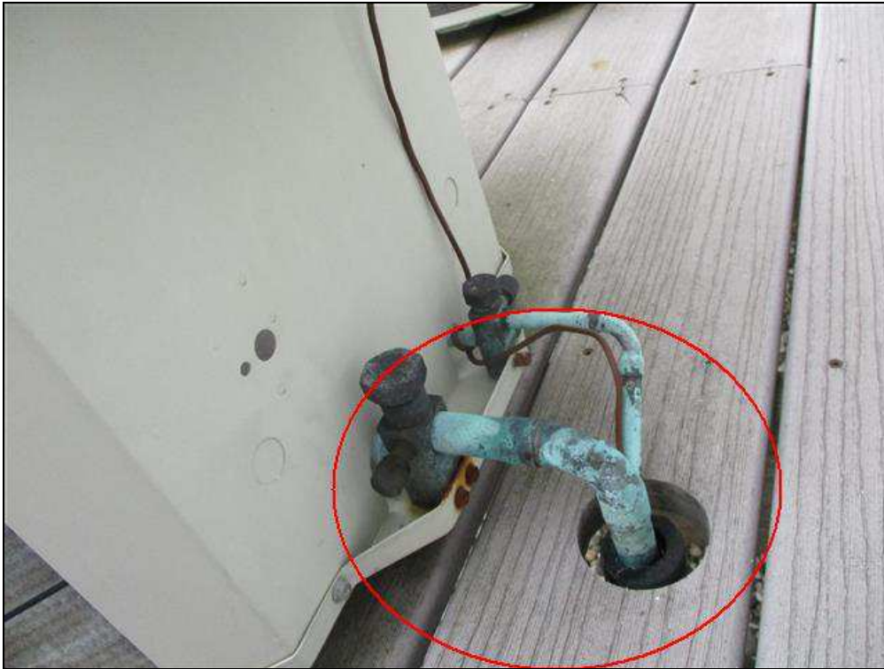
4.8 Item 2(Picture) Missing insulation
